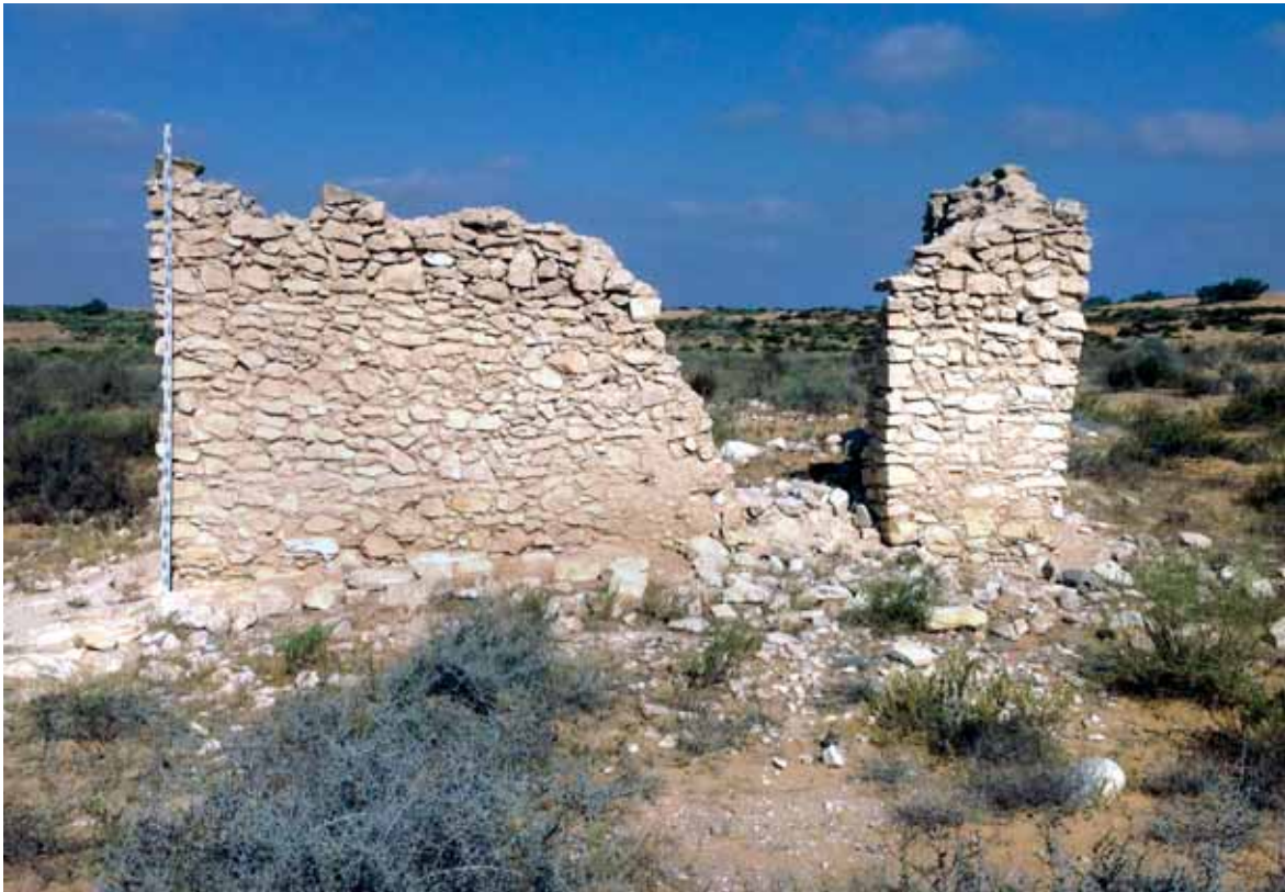
Fig. 8. Al-'Obeidat structure 4: view to the west; scale measures 3 m (photograph by B.A. Saidel)
