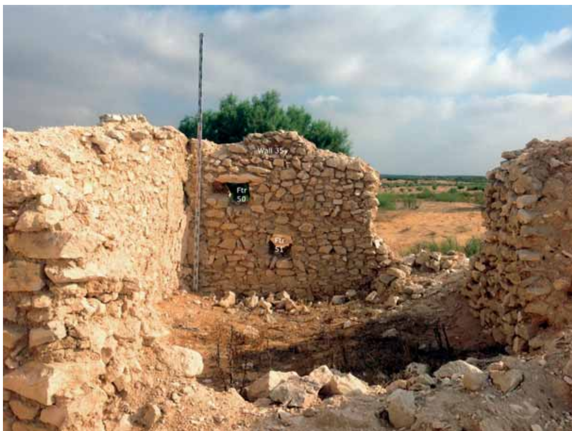
Fig. 6. Room A in al-‘Obeidat structure 3: view to the north; scale measures 3 m (photograph by B.A. Saidel)
